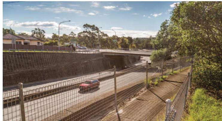
THE SITE IS ELEVATED ABOVE JAMES RUSE DRIVE AROUND ITS INTERSECTION WITH KISSING POINT RD
