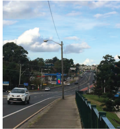
10B - VICTORIA ROAD CHARACTER (2): EAST OF RAILWAY LINE
